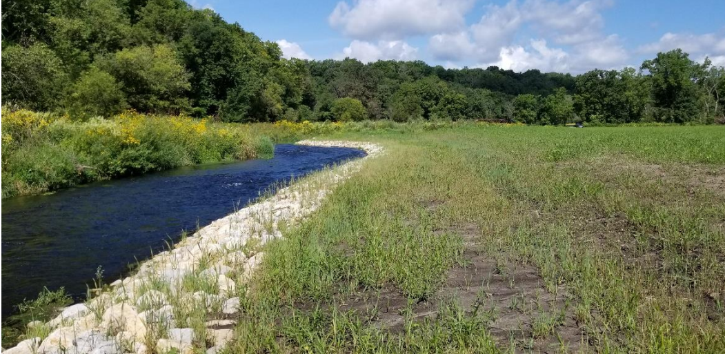
North Bear Creek on the Larson Farm in 2019, after streambank improvements.
